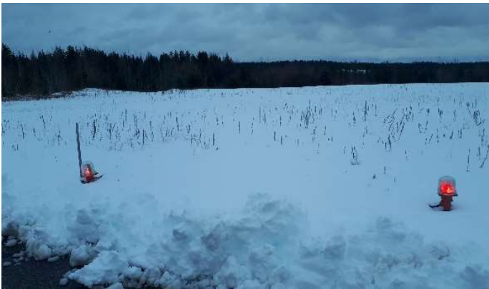
Figure 3-20 RWY 10-28 Threshold Lights
