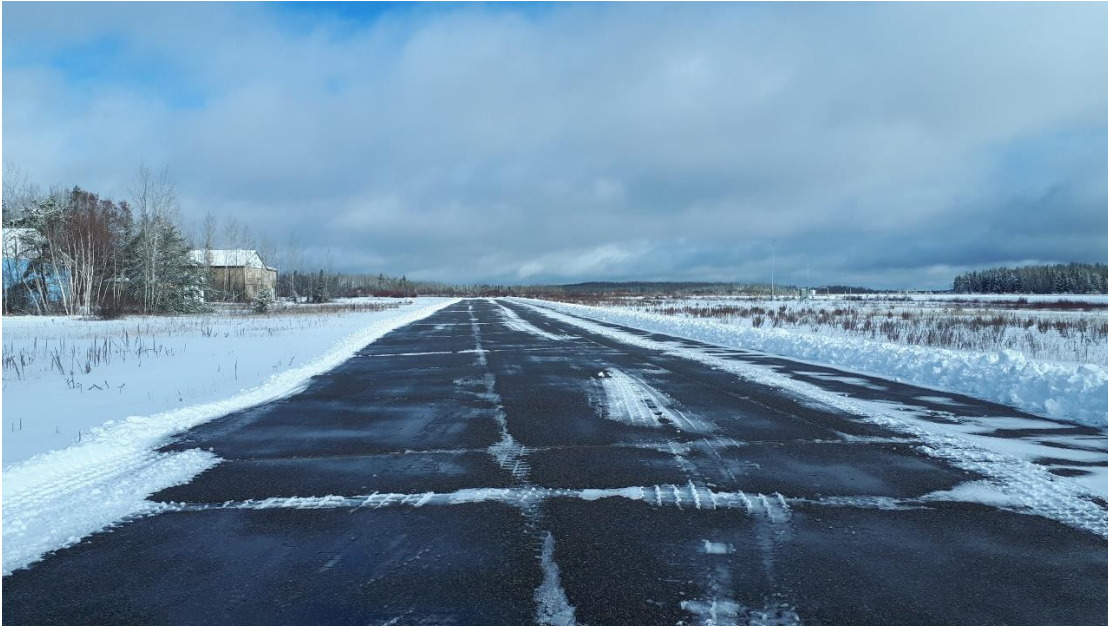
Taxiway to Hangars
