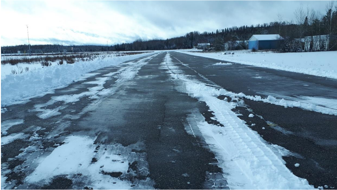
Taxiway to Hangars
