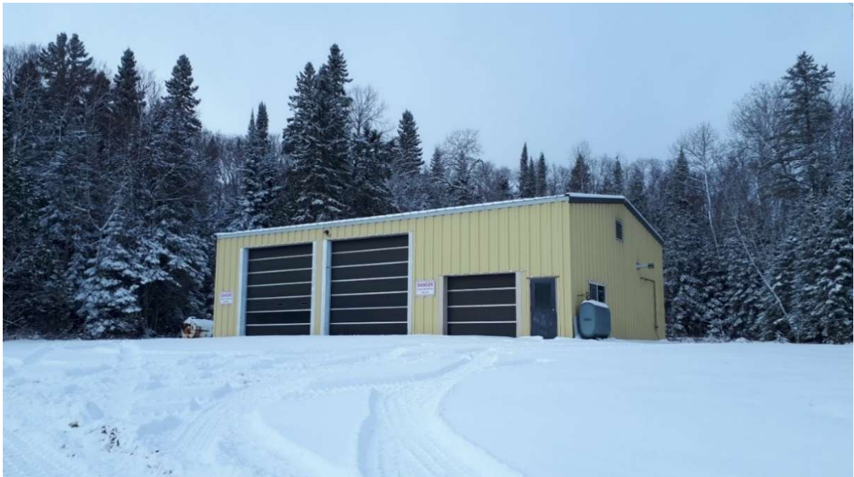
Figure 3-1 Maintenance Facility – View from Access Road
