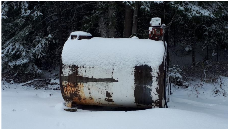
Fuel Tank for Maintenance Vehicles
