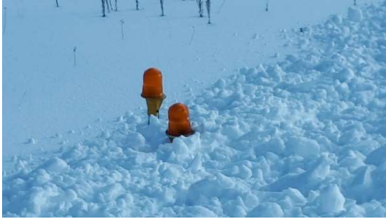
Figure 3-22 Apron – TWY Intersection Lights
