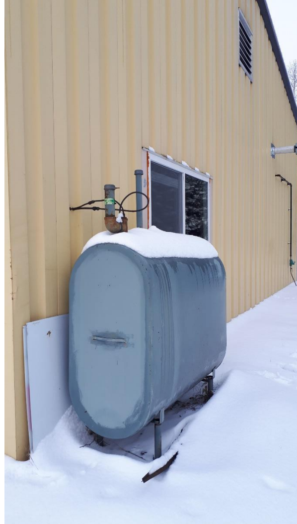
Maintenance Facility – Steel Tank for Fuel Oil and Lubricating Oil
