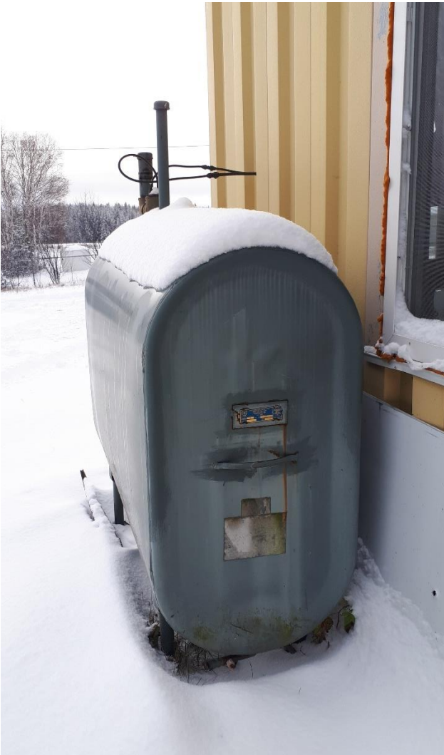
Maintenance Facility – Steel Tank for Fuel Oil and Lubricating Oil
