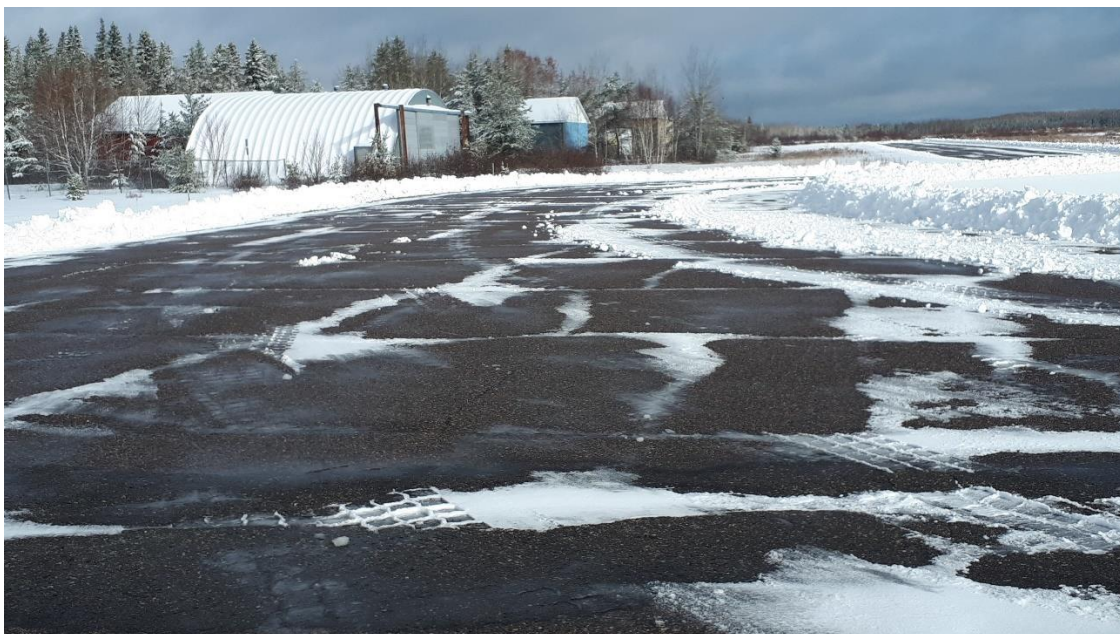
Taxiway to Hangars
