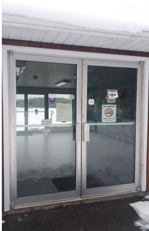
Access to Terminal Building Holding Room
