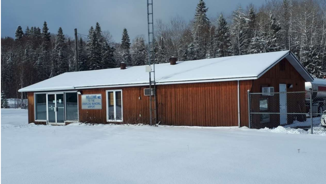
Figure 3-6 Terminal and Staff Offices Building - View from Apron
